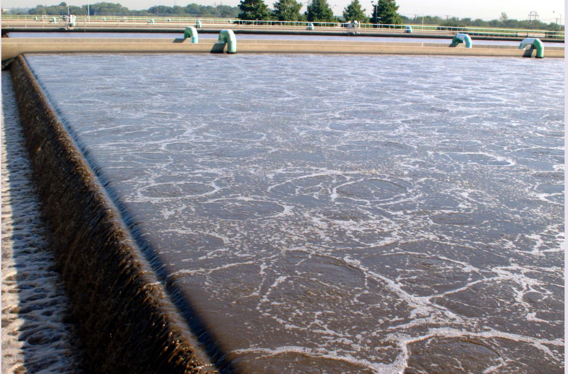
Treated Waste Water
